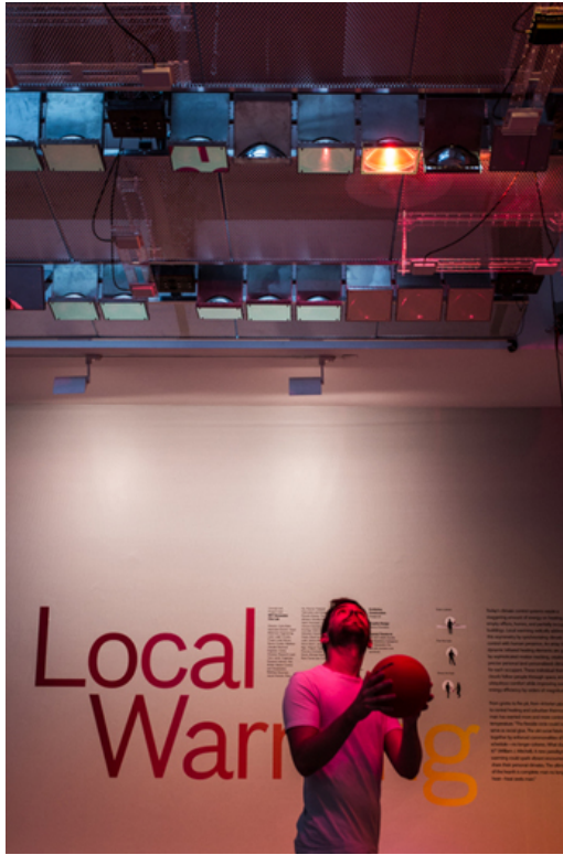
Infrared light beams follow occupants, creating personal climates. Photo: Aaron Nevin
