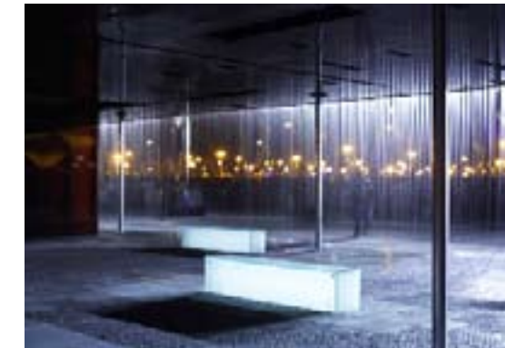
Digital Water Pavilion, Zaragoza, Spain, 2008 The 3,000 electromagnetic valves that control the water walls can be opened and closed to form a curtain of falling water with gaps at specified points. The result is an architecture that is fluid both literally and figuratively – a place where spaces are flexible, changing and responsive, and walls and doors can disappear and reappear.
